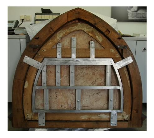
Fig. 5: Support metal construction on the back after the restoration in 2018. Photo:  $\mbox{\sc C}$  . Schneider.
