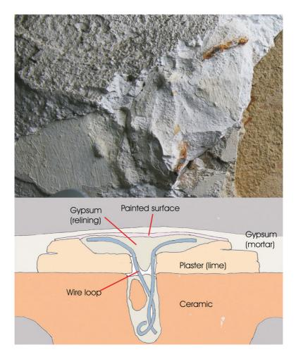
Fig. 11: Finding of the remains of lime plaster and the wire loop (top view) with schematic illustration of the stratigraphy (sectional view). Photo: © C. Schneider.
