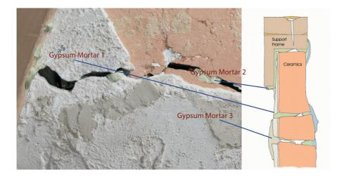
Fig. 8: Stratigraphy of the plaster mortar around the break joint (back). For better differentiation, the features in the picture on the left are coloured after the schematic drawing on the right. Photo: © C. Schneider.
